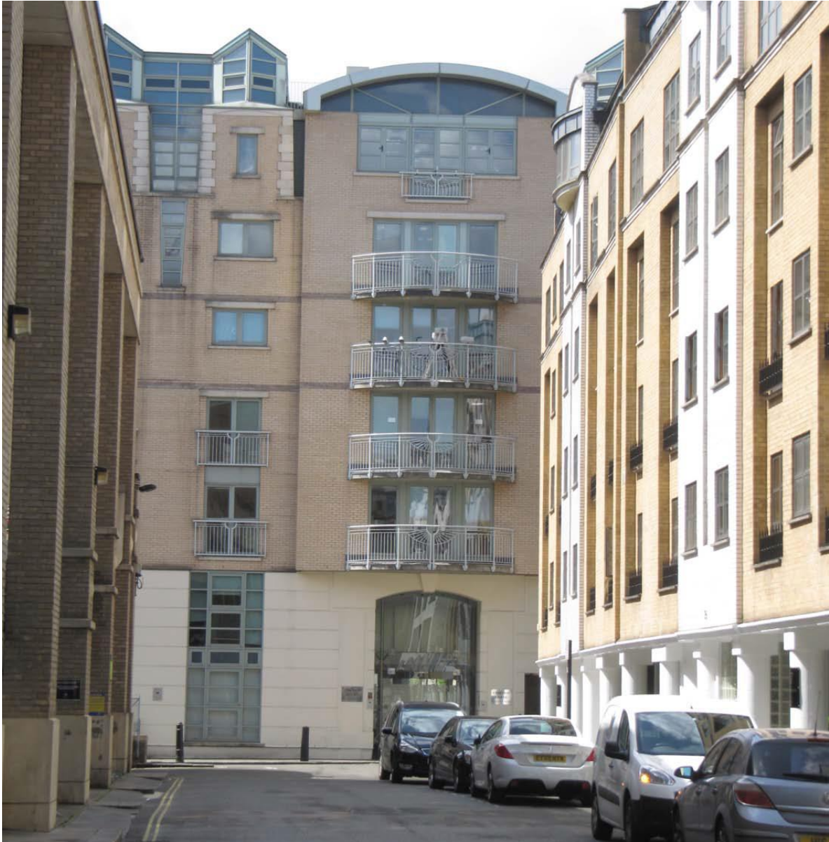
Redan Place View of Building
